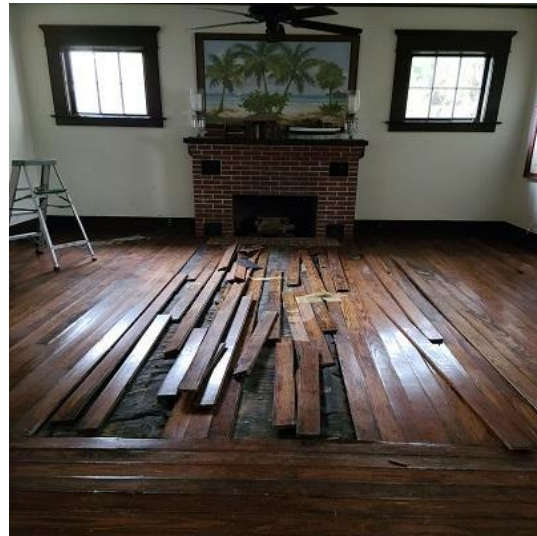
Beginning stages of restoration post Hurricane Ian
